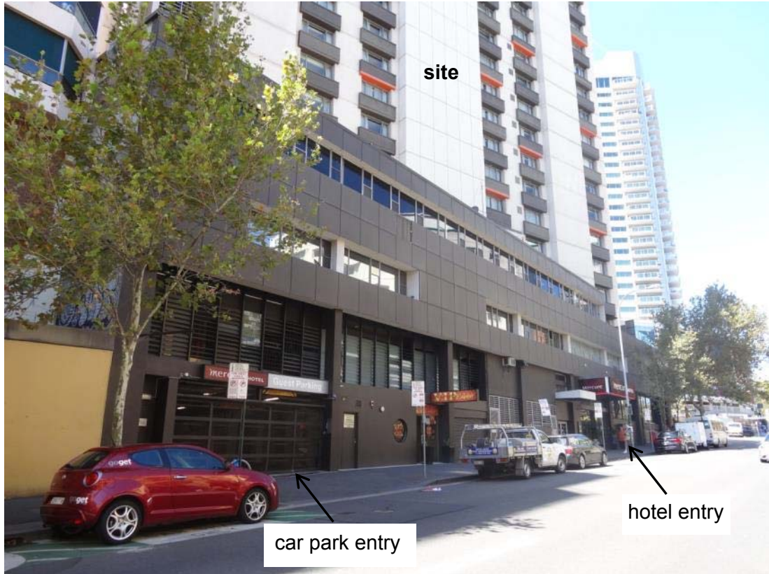
Figure 7: View of the Victoria Street facade (west) with a 3 storey podium containing entries to the basement car park, loading dock, and hotel foyer
