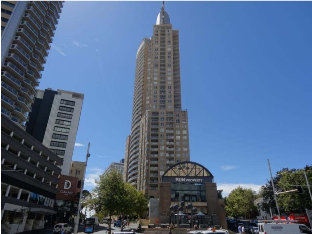
Figure 12: View of the Elan building at 1 Kings Cross Road, located to the south east of the site
