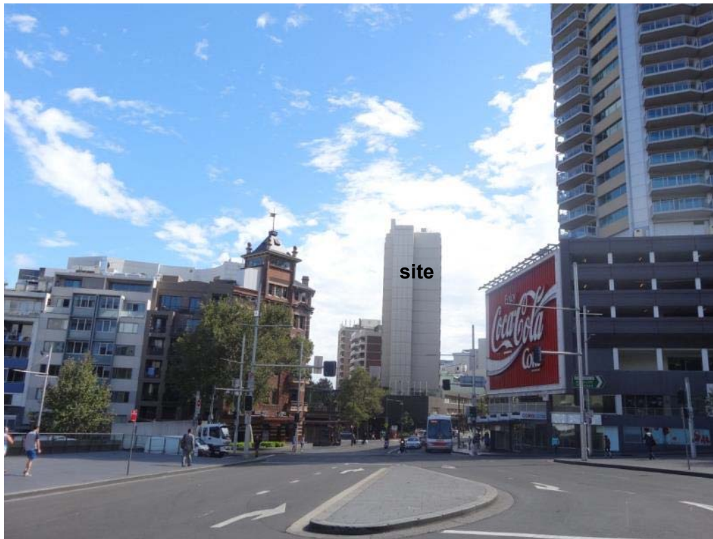
Figure 3: View of the site looking north-east from Victoria Street
