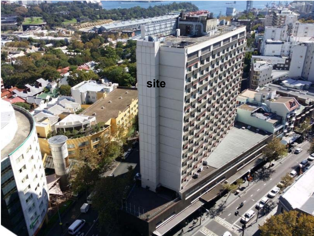
Figure 4: View of the site from adjacent residential tower located to the south, showing the plant room, and associated services located on the roof
