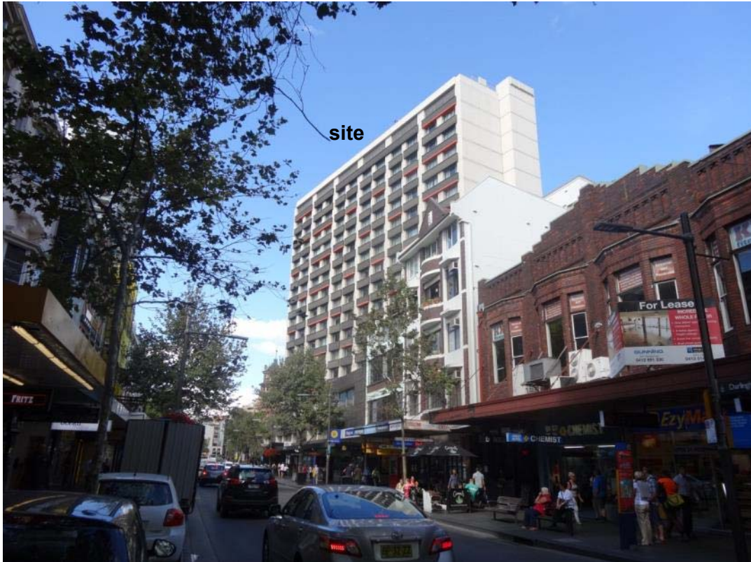
Figure 6: View of the site looking south west along Darlinghurst Road
